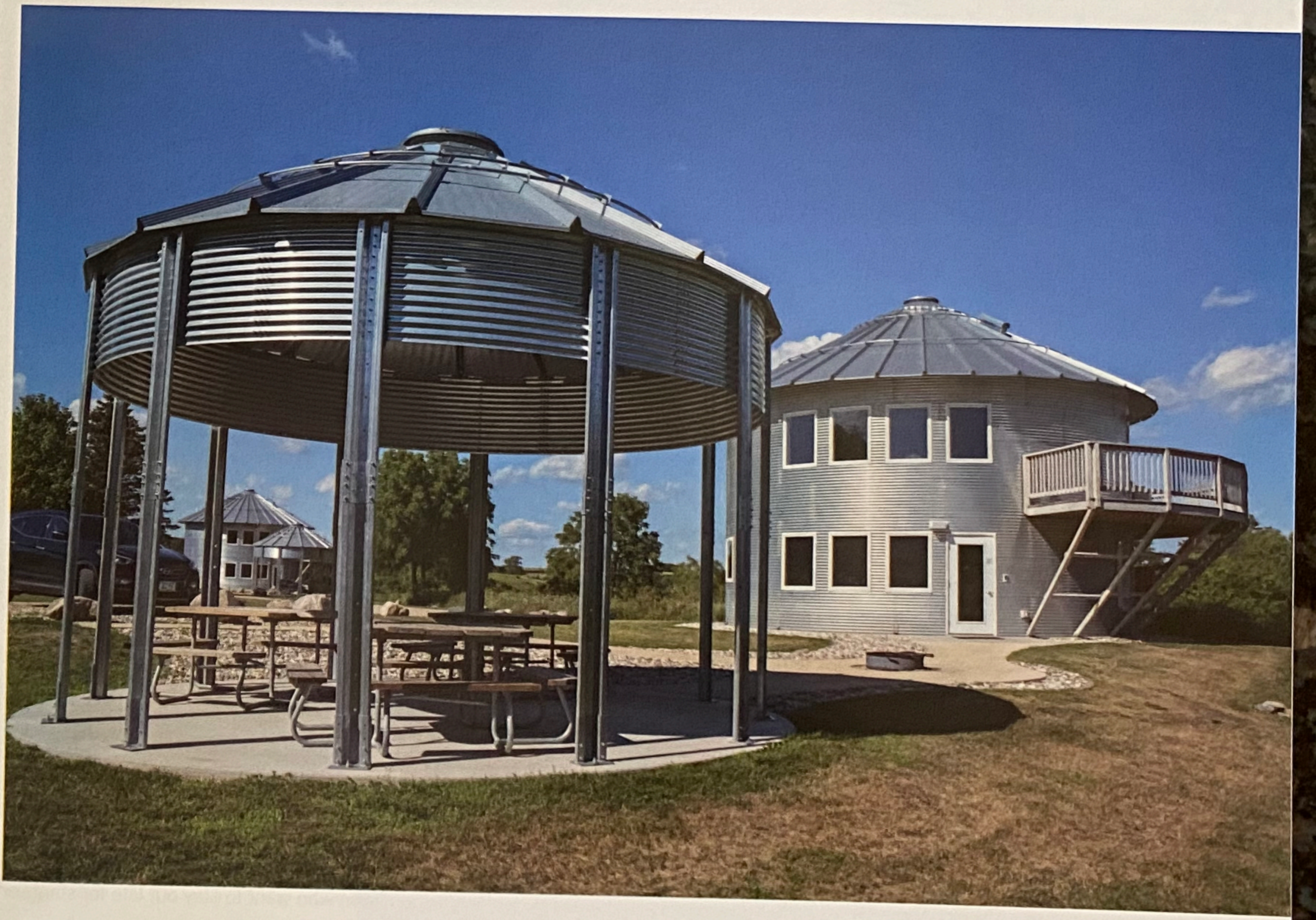
Below: Outdoor gathering areas and fire rings are connected to the cabins by paved walkways.
