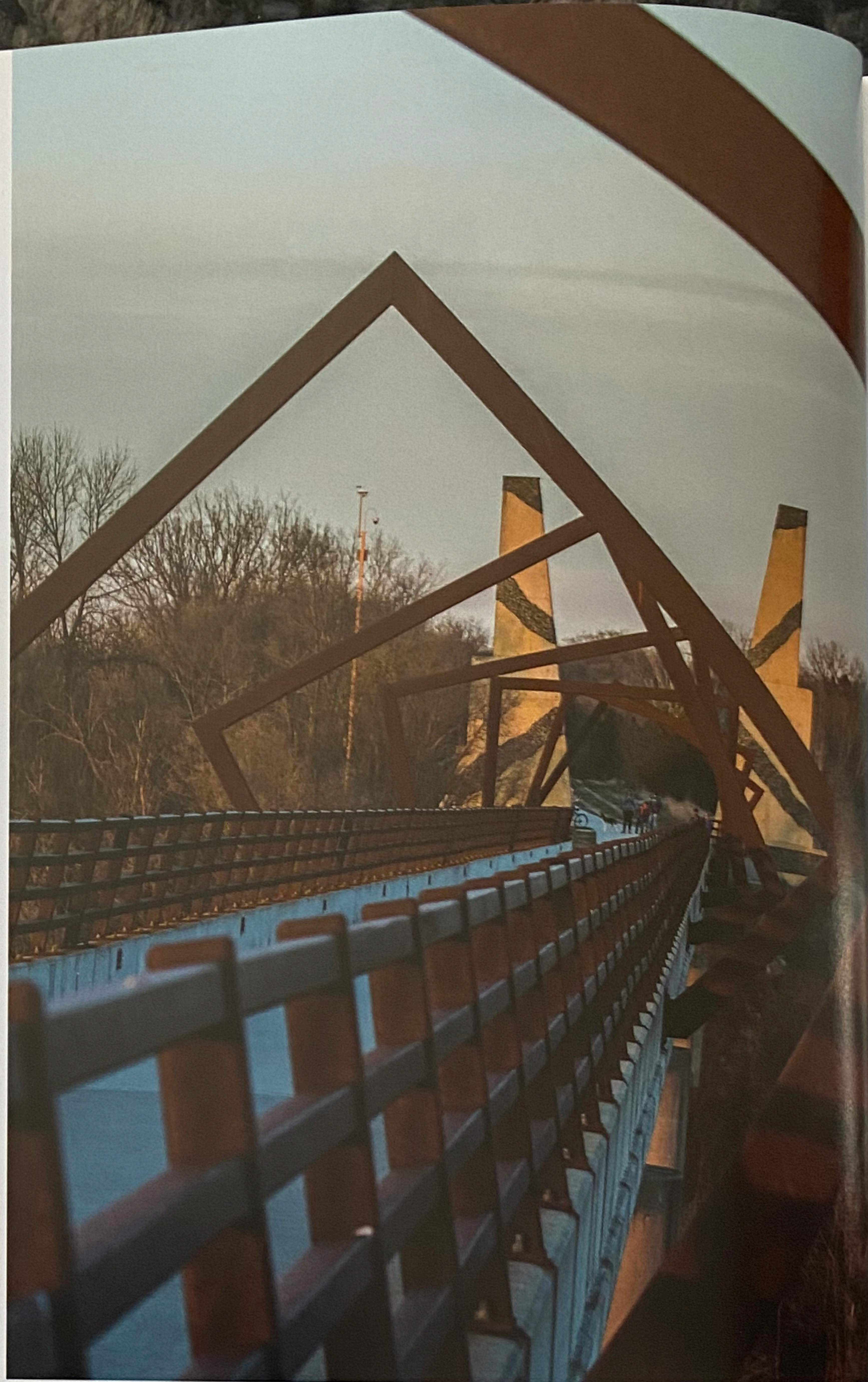
Above: The High Trestle Trail bridge is the highlight of a 25-mile trail that spans four Iowa counties. It was built atop existing 130-foot-tall piers previously owned and used by the Union Pacific railroad. Photo by Brian Abeling.
